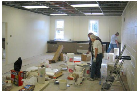
One of the many rooms that were painted.
